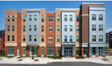
South Pointe Commons Clark-Metro $12 Million
