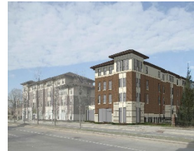
Greenbridge II Midtown $11.1 Million Opening 2018
